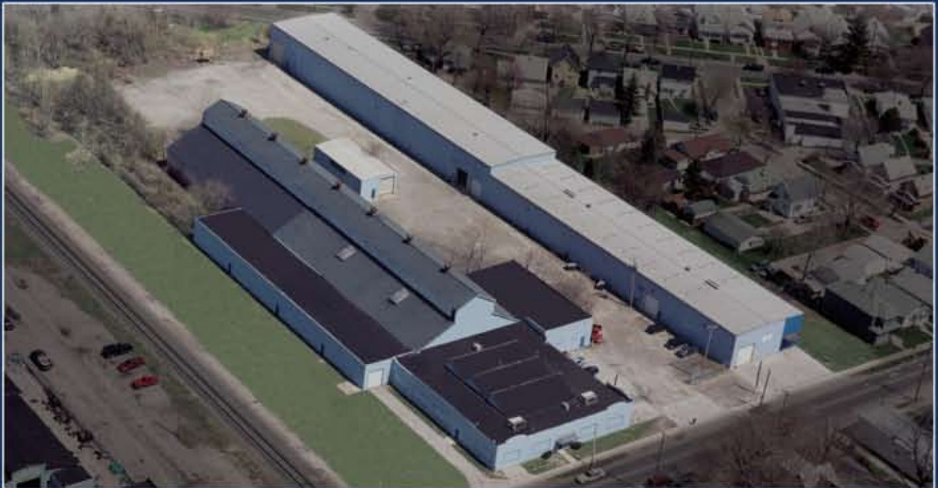
Parker Steel's Toledo, Ohio Warehouse
